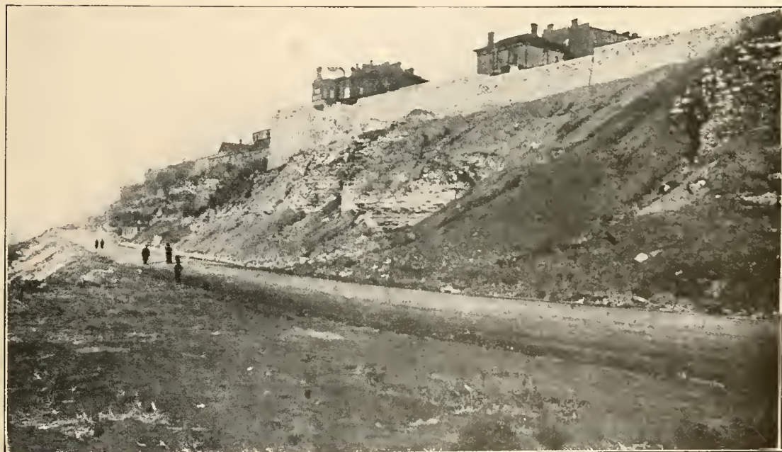
KERSEY COATES TERRACE, AFTER GRADING.
